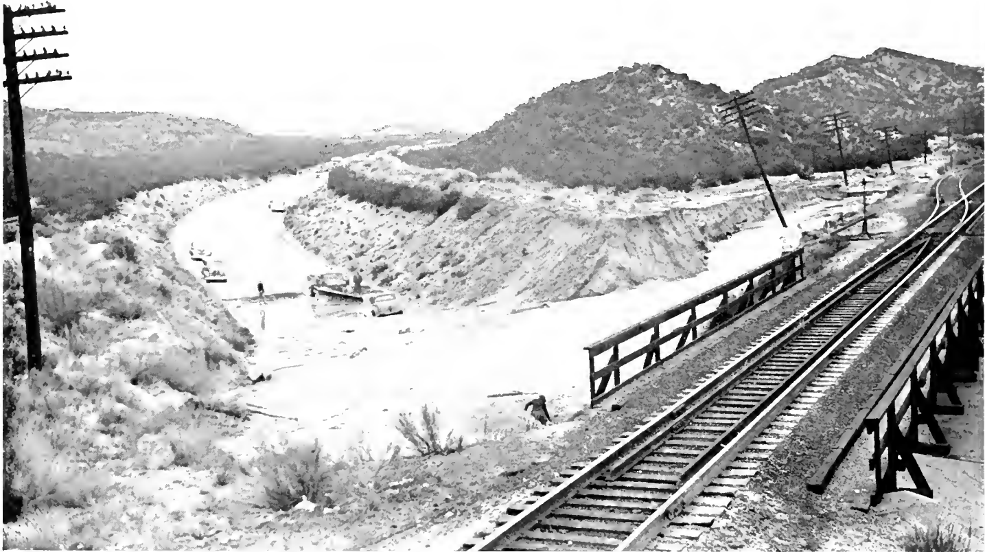
U. S. 66 blocked by flood debris at railroad underpass near Gish, San Bernardino County. Railroad was also washed out
